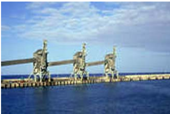
Bridgetown—Conspicuous Sugar-loading Towers
