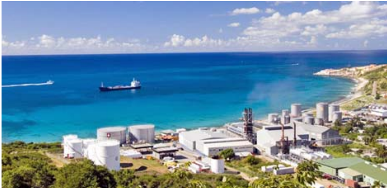
Cole Bay Oil Terminal
