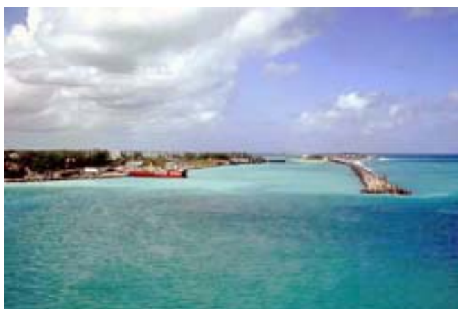
Arawak Cay—West Breakwater
